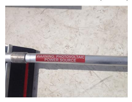
Disconnects on the exterior of the building prior to the Ameren power source shall be clearly labeled. For inverters installed in the building interior, reference to the location of the disconnect shall be provided at the meter and at the inverters.
