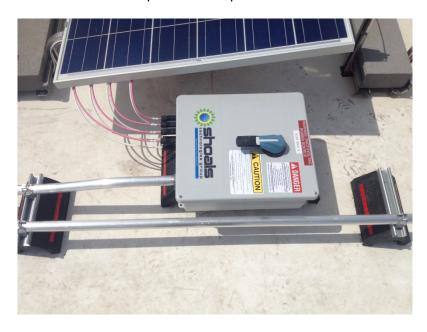
Exterior wiring must be placed in enclosed conduit. Conduit shall be labeled every 10 feet and within 1 foot of turns or bends and within 1 foot above and below penetrations per IFC 2021
