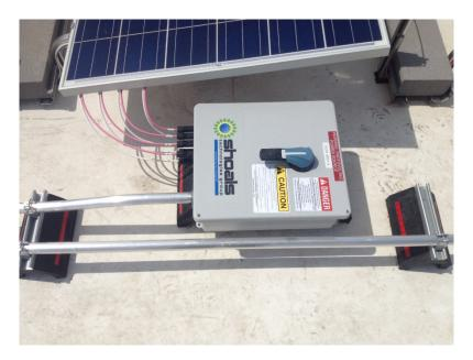
Exterior wiring must be placed in enclosed conduit. Conduit shall be labeled every 10 feet and within 1 foot of turns or bends and within 1 foot above and below penetrations per IFC 2018
