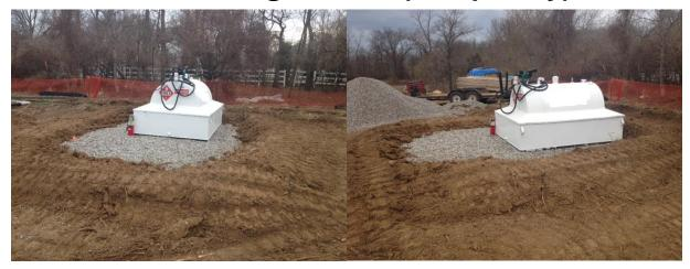
A permit is required for the placement and use of any fuel storage tank exceeding 50 gallons liquid capacity. The tank must be installed, operated and maintained in accordance with IFC 2012 Chapter 57.
